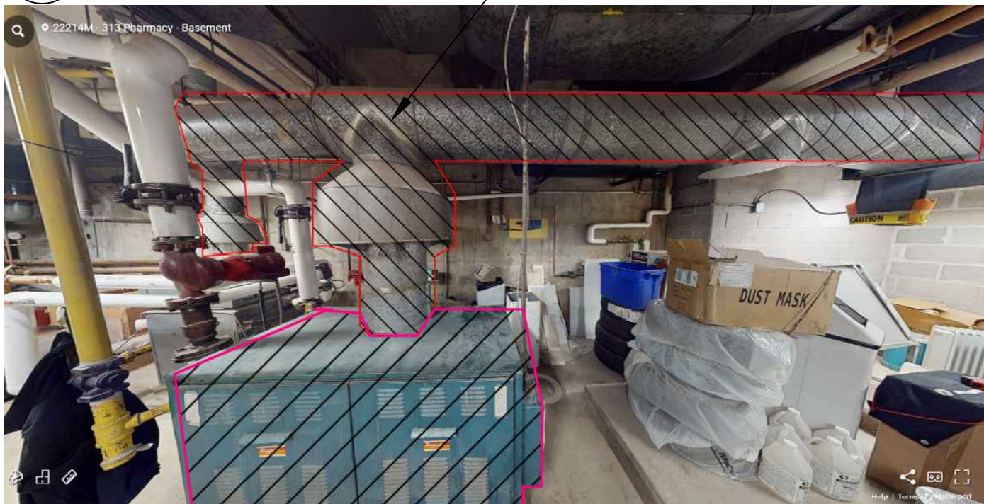
5 DEMOLITION OF POOL WATER BOILER MD-01
