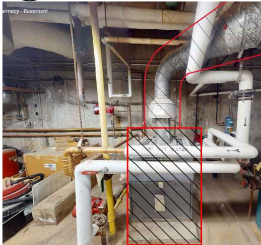
3 DEMOLITION OF HEATING WATER BOILER MD-01
