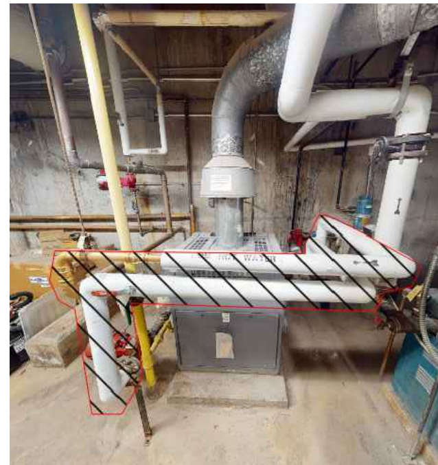
3 DEMOLITION OF HEATING WATER BOILER PIPING MD-02
